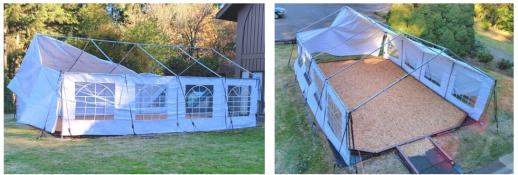
With help from Dick Eyberg, Mike Barth, Clay Morgan, Dave Tomastik and Dennis Zerba, the roof canvas was pulled back into place. New grommets were installed to replace the ones pulled out and additional grommets and other tiedowns were installed to help prevent similar incidents in the future.
